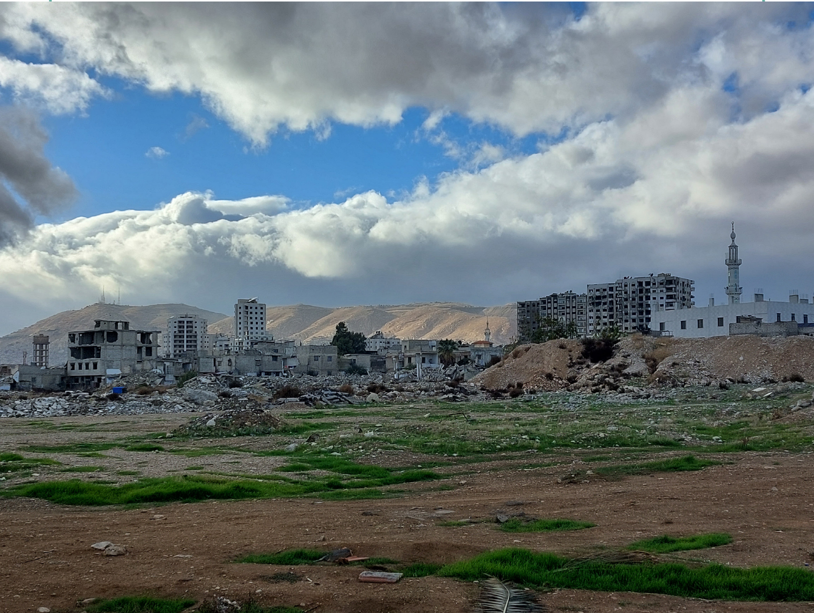
Destroyed buildings in Harasta, Rif Dimashq ©Damascus Voice
